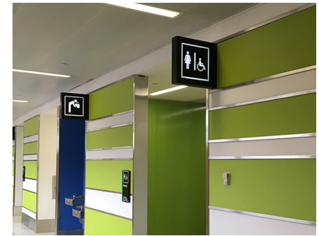
Overhead signs oriented in the direction of travel provided in addition to required Braille signs.
