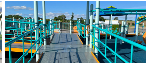
Ramps have a low slope and handrails are at children's height.
