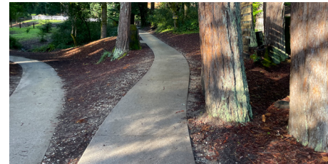
Small compacted crushed rock (left) and concrete (right) are both good surfaces with proper ground prep.
