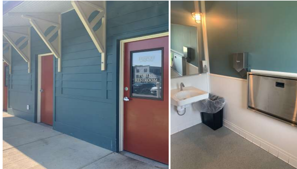
These single-occupancy permanent restrooms were clean, functional, and well maintained. They were designed to maximize accessibility for all users. (Fairport)
