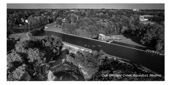
The basin in Medina, with its L shape and straight lines, was built as part of the Barge Canal enlargement of 1905 through 1918. An aqueduct carries the canal about 70 feet above the Old Orchard Creek, which flows south to north and ends at Lake Ontario. This is the only aqueduct on the Barge Canal. The creek drops over Medina Falls just to the north of the canal, then runs into man-made Glenwood Lake.
