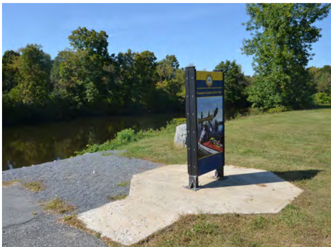
Simple bank launch sites can be highly effective, but designers should be careful to specify a surface type that is durable, stable, and erosion resistant. Fine stone may become washed away if not stabilized in some way. (Fort Miller)
