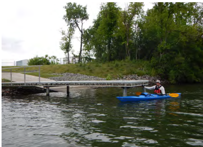
Boarding or high-freeboard docks at boat ramps are often too far above the water to be of use to paddlers, but enhancements such low-level boarding planks or floating dock extensions can be added to improve the situation.
