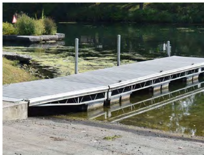
Gangways and floating docks are also used as boarding ramps at trailer launch sites. They are usually designed with higher freeboard to allow boarding of powerboats. (Seneca Falls Boat Ramp, Cayuga- Seneca Canal)
