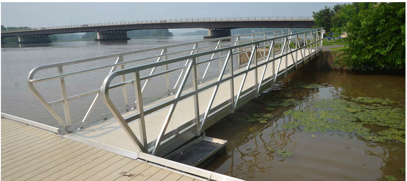
Gangways allow for a transition between a fixed abutment on land and a floating dock that moves with changes in water level. Most gangways require additional flotation at the dock end to maintain a level dock surface.(Crescent)
