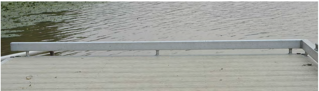
Edge protection is important for the safety of wheelchair users and can also serve as a grab rail and temporary mooring point installed atop short posts.
