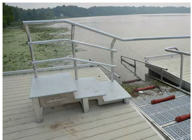
Transfer benches can be added to docks with launch slides to allow easier entry for wheelchair users. Grab rails help all paddlers enter and exit watercraft.
