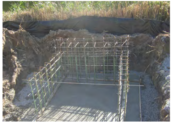
Gangways and structural arms that connect floating docks to land require firm shore-side abutments, deadmen, or piers. These are large, heavy structures that should be sized and designed by a professional. (Onondaga Lake Outlet, Liverpool)
