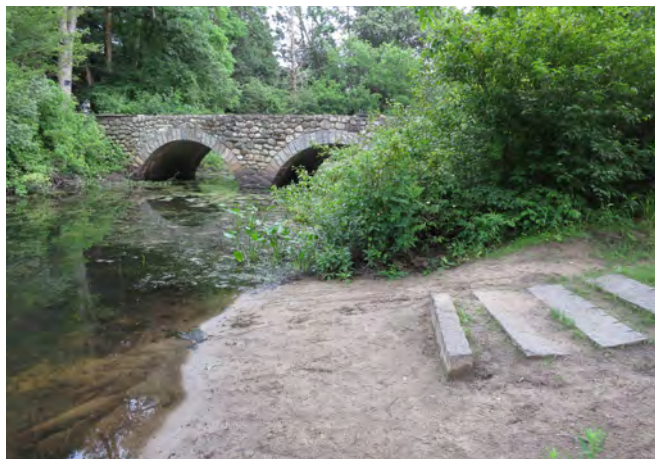
Wide steps made of stone or concrete can ease the grade transition for bank launches and reduce erosion. (Wellesley, MA)
