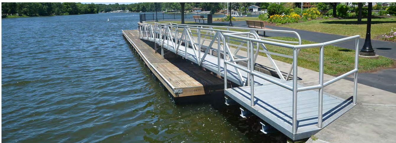
Floating docks can have a narrow protrusion in to the waterway when fitted with a landing and gangway parallel to the shore. (Papermill Island, Baldwinsville)
