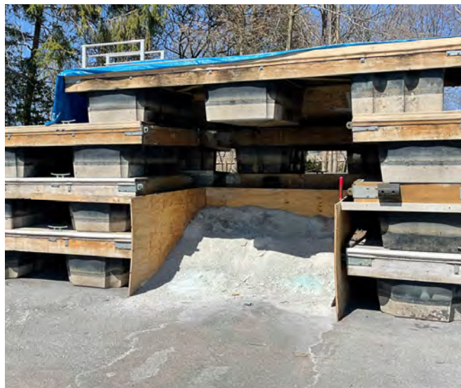
Safe storage of docks which require seasonal removal is an important operational consideration for designers. This dock storage site in Baldwinville doubles as road salt storage.
