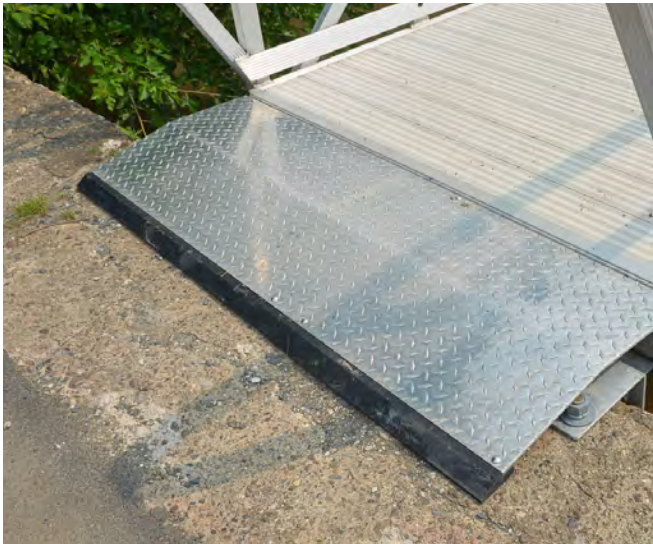
Transition plates allow for a smooth transfer on and off the gangway, bridging over potential obstruction or trip hazards. A replaceable wear edge protects the plate from abrasion.
