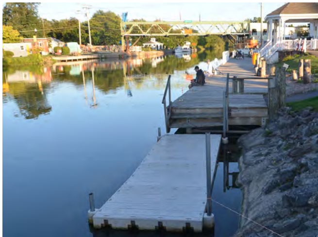
A floating dock can enhance the utility of an existing high-freeboard dock for paddlers but steps will be a barrier to some users. (Spencerport)
