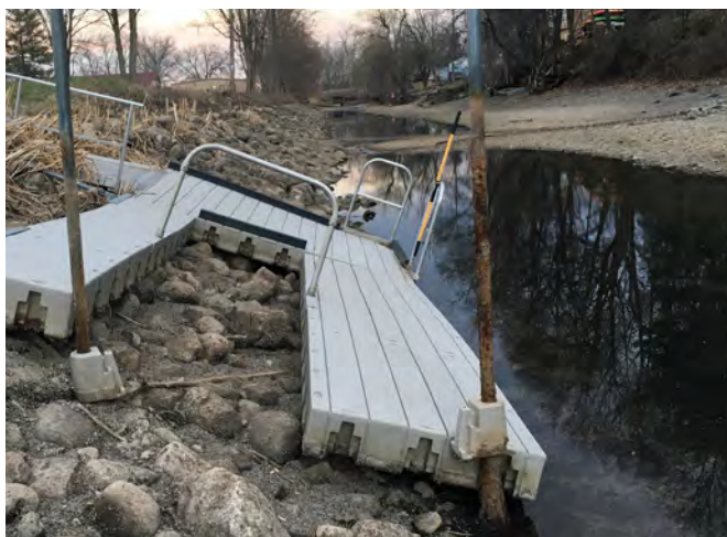
Winter drawdowns can place enormous stress on dock and launch components.
