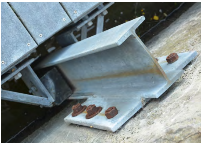
Heavy duty hardware like these slides and rails used on shore anchors will stand up to the rigors of the canal much better than lightweight equipment. (Medina)
