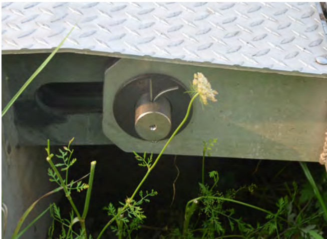
Designers should specify rigid or semi-rigid connectors between dock sections to provide stability underfoot with hinged or rolling connections on gangways to accommodate fluctuating water levels. (Freeman's Bridge, Glenville)
