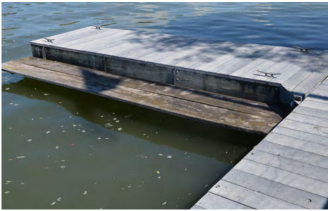
Low freeboard extensions can be added to floating docks to improve paddler access (Medina).
