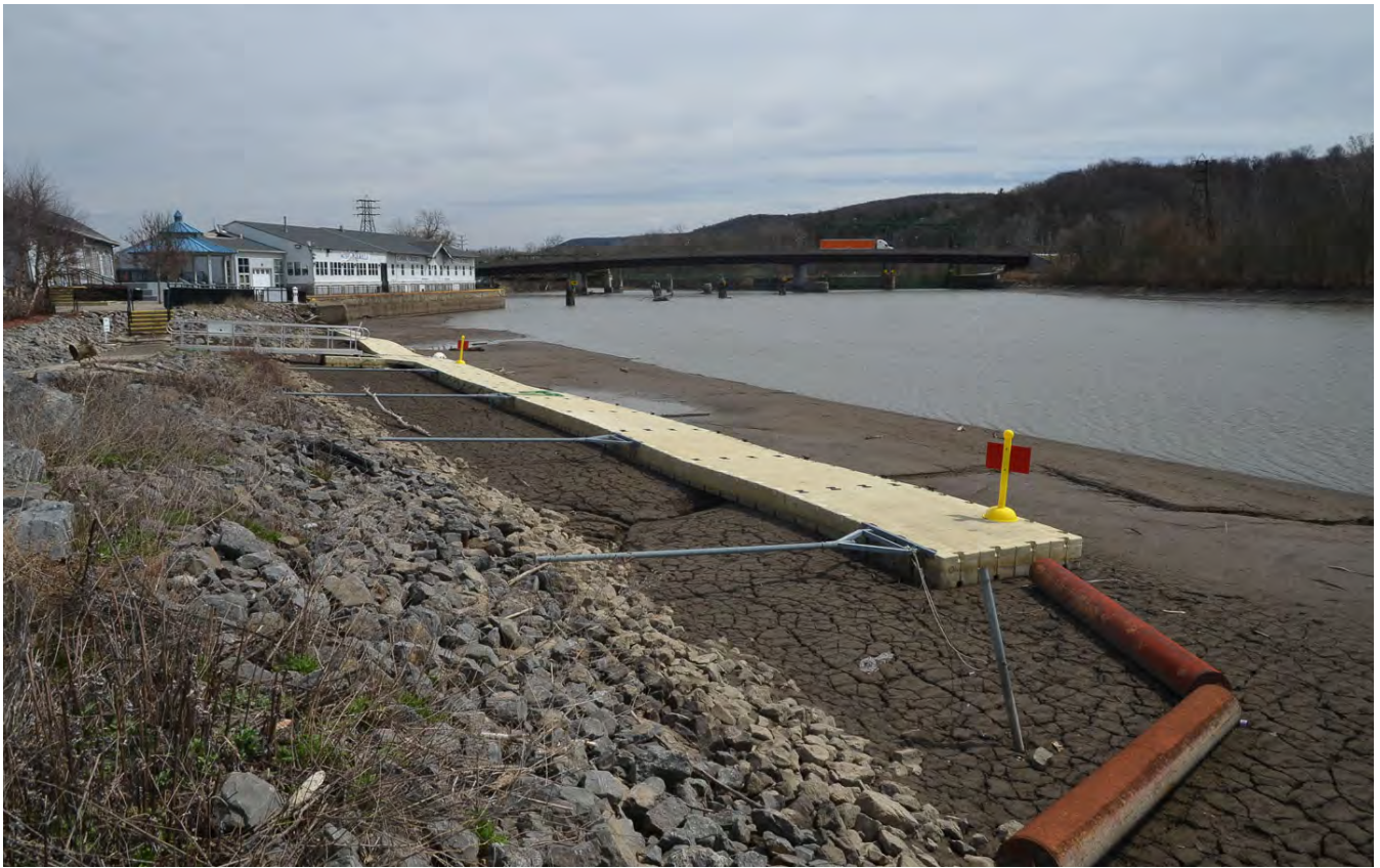
Designers need to consider what happens to docks during low (or no) water conditions. This floating dock rests on a flat shallow bottom during the winter, but that is not the case in all locations. (Herkimer)
