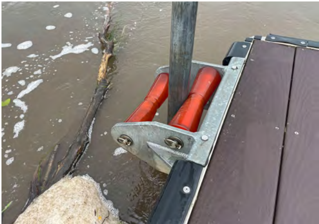
Pile guides are essential hardware that allow pile anchored floating docks to move up and down with water level changes. They are offered in several styles.
