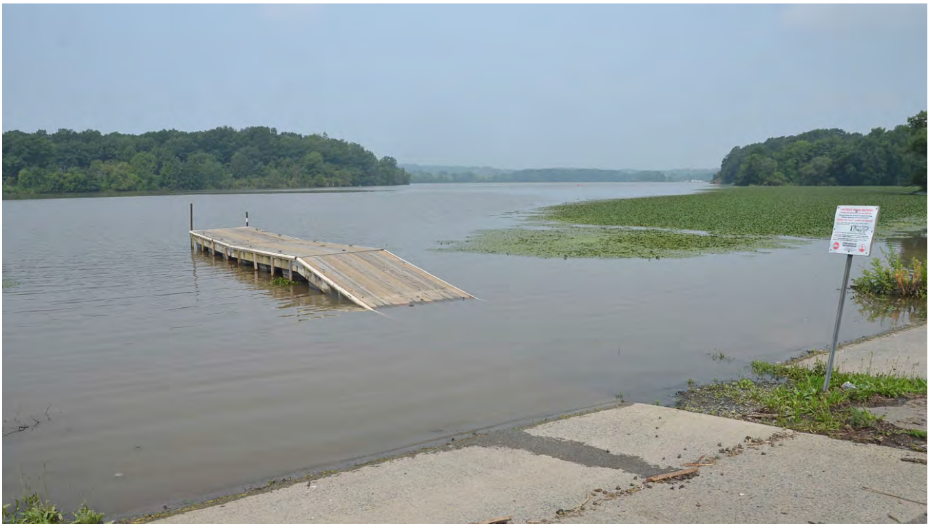
High water can render launch facilities like this ramp and floating dock unusable at times. Designs should take into account the increased frequency of flooding events. (Waterford)
