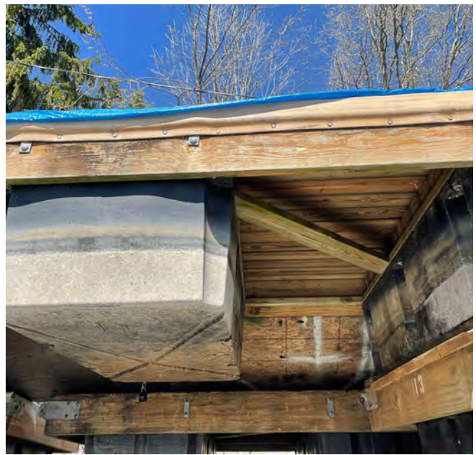
Flotation for docks is often provided in the form of purpose-built plastic float chambers which are designed with attachment points. The spacing and sizing of these floats will have an impact on freeboard and stability and should be designed by a professional with experience in these calculations.
