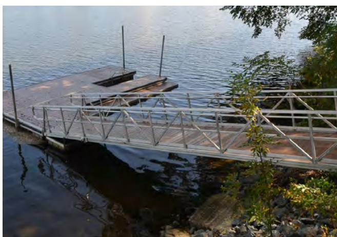
Floating docks may require long gangways, depending on the elevation of the shoreline and the amount of water level fluctuation during the navigation season. Designers should consider land grading to reduce the required length of gangway. (Lighthouse Park, Champlain Canal/Hudson River, Halfmoon)
