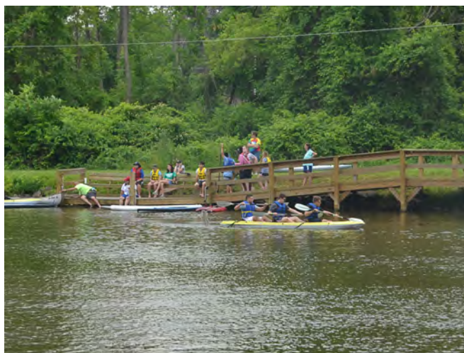
Fixed docks are more stable than floating docks, but may have higher freeboard, or be flooded by high water levels. This one works for canoes and stand-up paddleboards but may be more difficult for kayaks. At lower water levels, they may become unusable. (SUNY Brockport)
