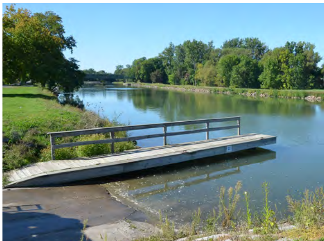
A trailer launch with a fixed boarding pier is typical of ramps found on land-cut portions of the Canal System. (Albion)
