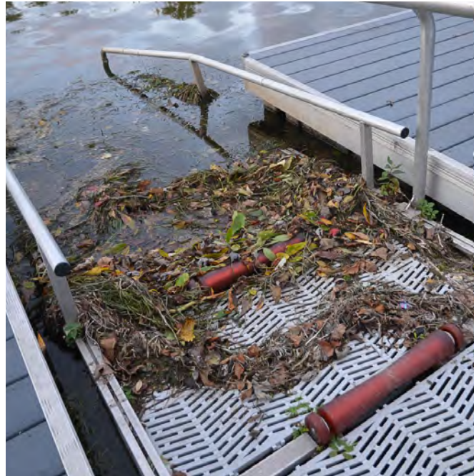
Floating debris can affect the functioning of launch components.
